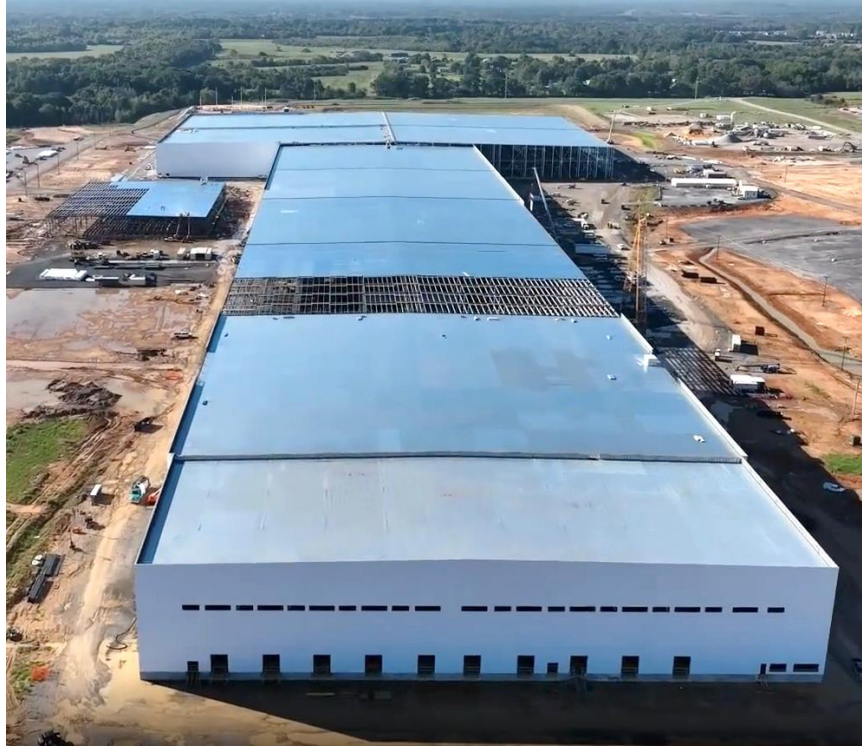
Amplify Cell Technologies Battery Factory, Byhalia, MS
