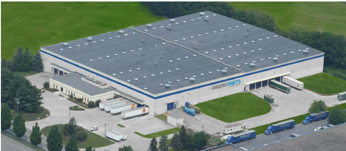
PACCAR's Parts Distribution Center in Lancaster, Pennsylvania
